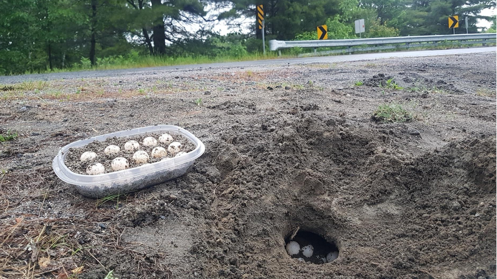
Turtle eggs collected during road construction will be incubated offsite. Photo: Kayla Martin/GBB
